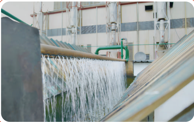
Water Treatment Plant (WTP)
