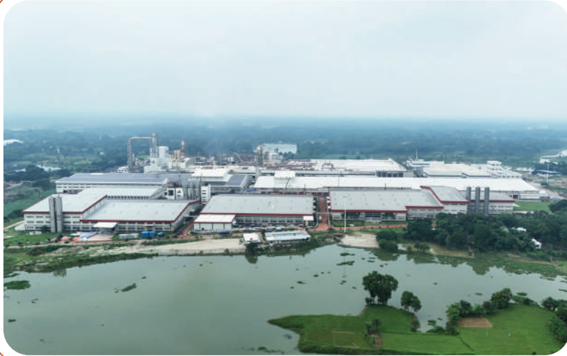
Factory and Factory Riverside (Green Policy)
